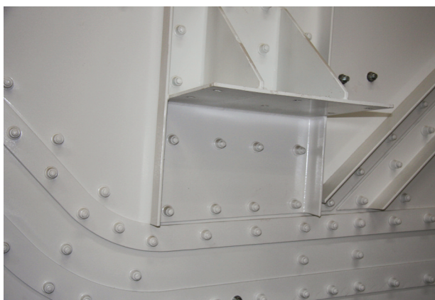
All steel plates are weldless and are assembled using Huck-bolts, to reduce stress on the structure.
